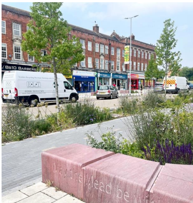
Above: This 'high performance' tree pits on Arnside Road, in Southmead, Bristol, combines the use of structural soil (Stockholm System), sustainable urban drainage and wildlife-friendly underplanting alongside a new cycle route to deliver multiple benefits. Image: Ben Rose.
